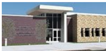
Aspen Drive Branch Library, Vernon Hills
